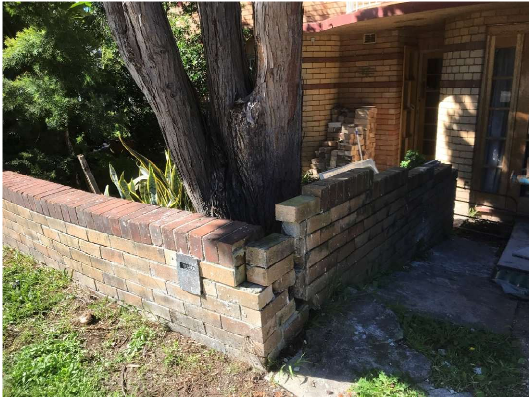
Image 5: The base of the Cyprus tree illustrating the damage to the brick fence and driveway
