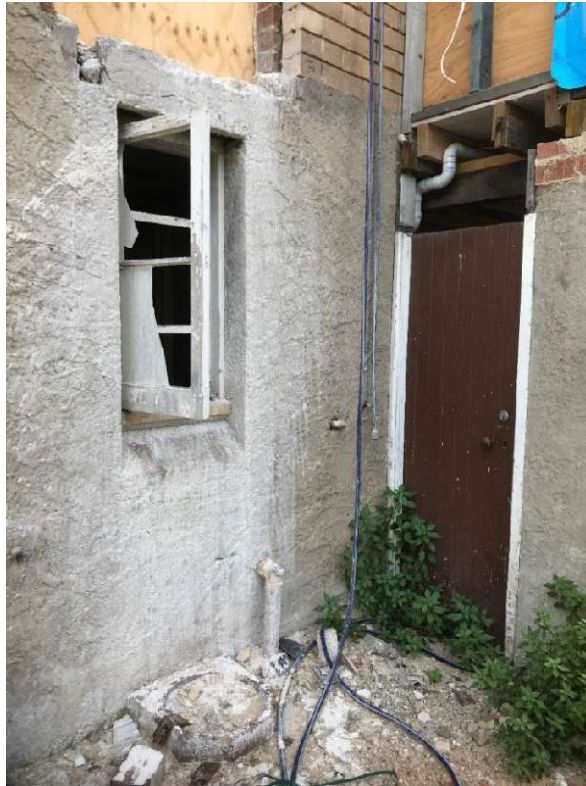
Image 15: The damaged laundry window proposed to be replaced.
