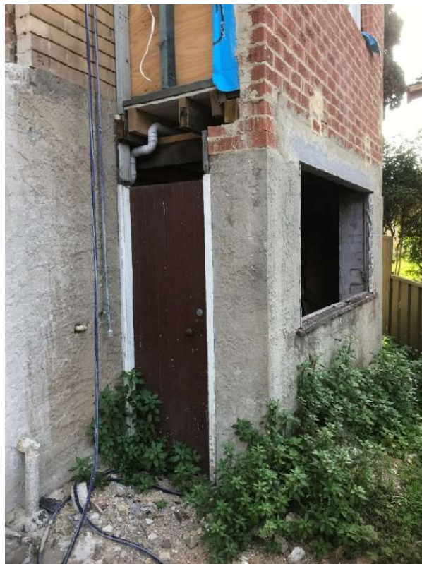
Image 16: The basement window proposed to be partially cut down to form a door with a side light window
